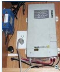
We are delighted that our batteries are being kept in good condition with the help of the TRUECharge2. At \$120 per battery, we want to keep them for a while and harvest the maximum number of amps per charge that we can. If we were using AGM batteries, this charger would be a hands-down must-add for the motorhome, because of its smart charging characteristics. Regardless of the batteries used, the Xantrex TRUECharge2 represents the ultimate in onboard vehicle battery charging.
